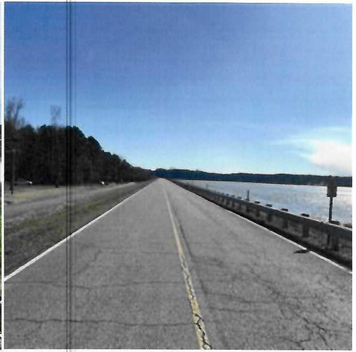
PHOTO 6—Dam crest view from left side of dam
