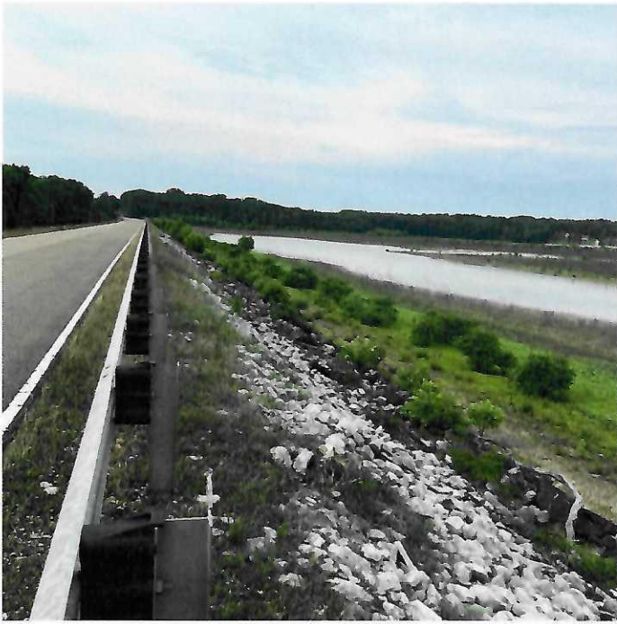
PHOTO 5—Upstream slope view from left side of dam
