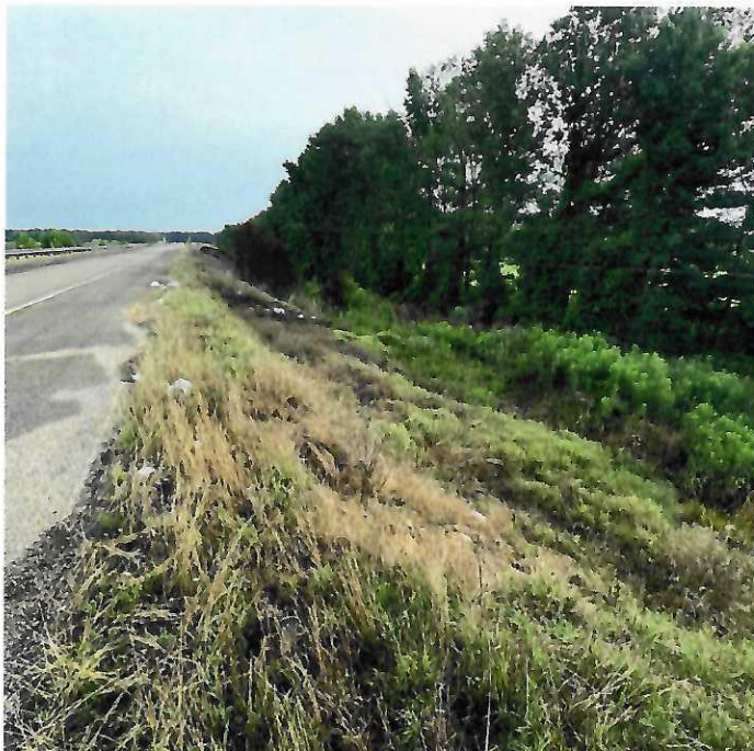
PHOTO 3 —Downstream slope view from right side of dam
