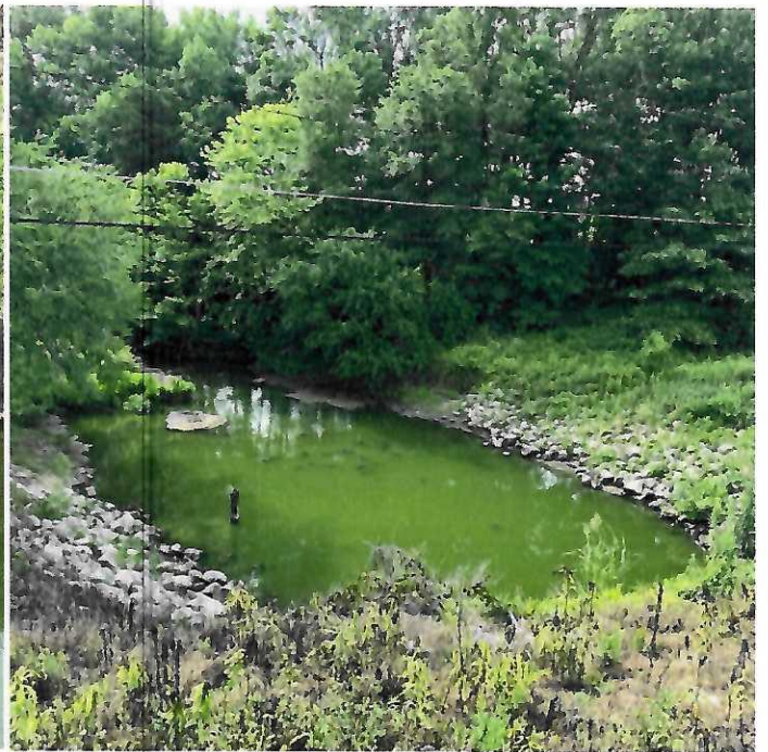
PHOTO 10—Exit channel view from end of outlet structures
