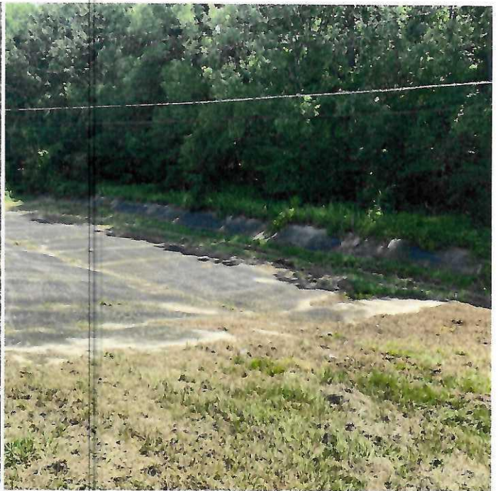
PHOTO 14— Bottom of auxiliary spillway
