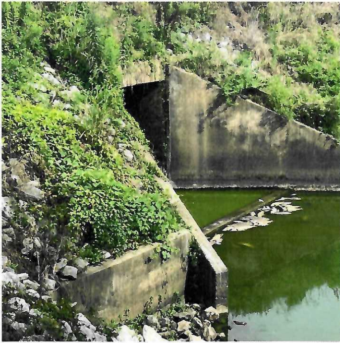
PHOTO 9—Spillway outlet structures from front view
