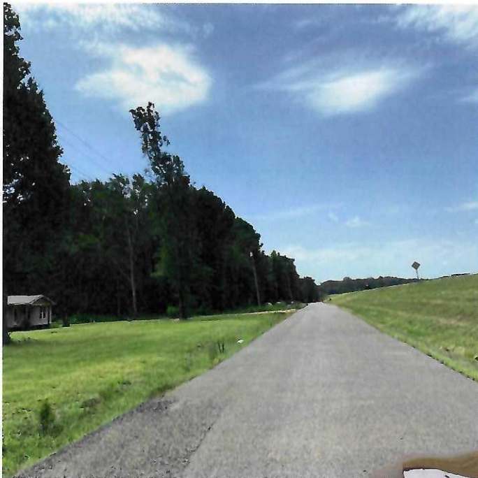
PHOTO 15 — Utility lines along Perkins Road
