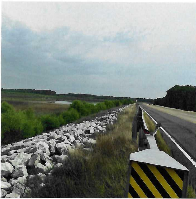
PHOTO 1—Upstream slope view from right side of dam
