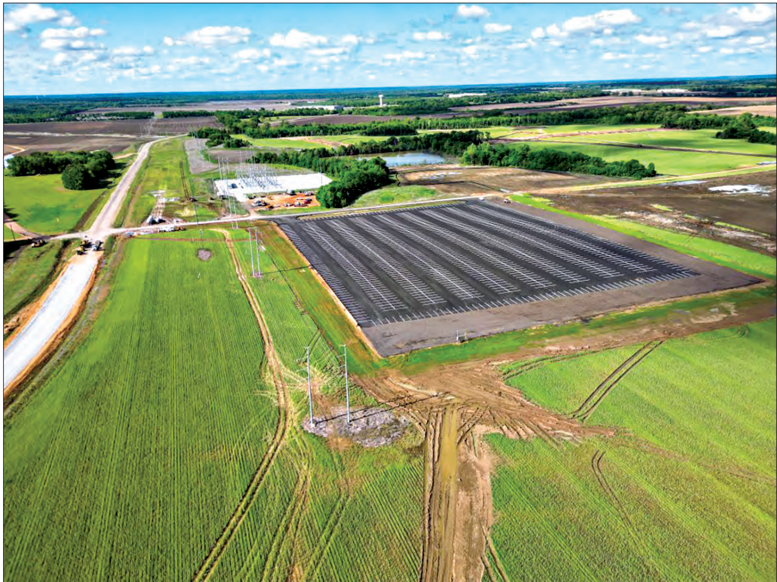
The future Aluminum Dynamics Inc. at the Infinity Megasite is shown in this aerial photograph. This Megasite is one of three in Lowndes County. Now, the Golden Triangle Development LINK and Lowndes County Board of Supervisors are working to find and work toward the next one, Cinco.
